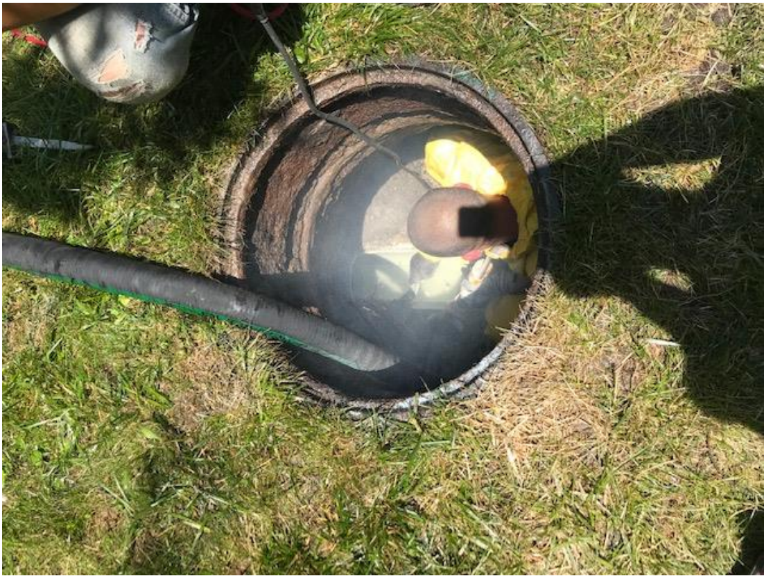
Open-cut point repair, replaced 5.5' of 10" clay pipe with SDR 35 PVC pipe
