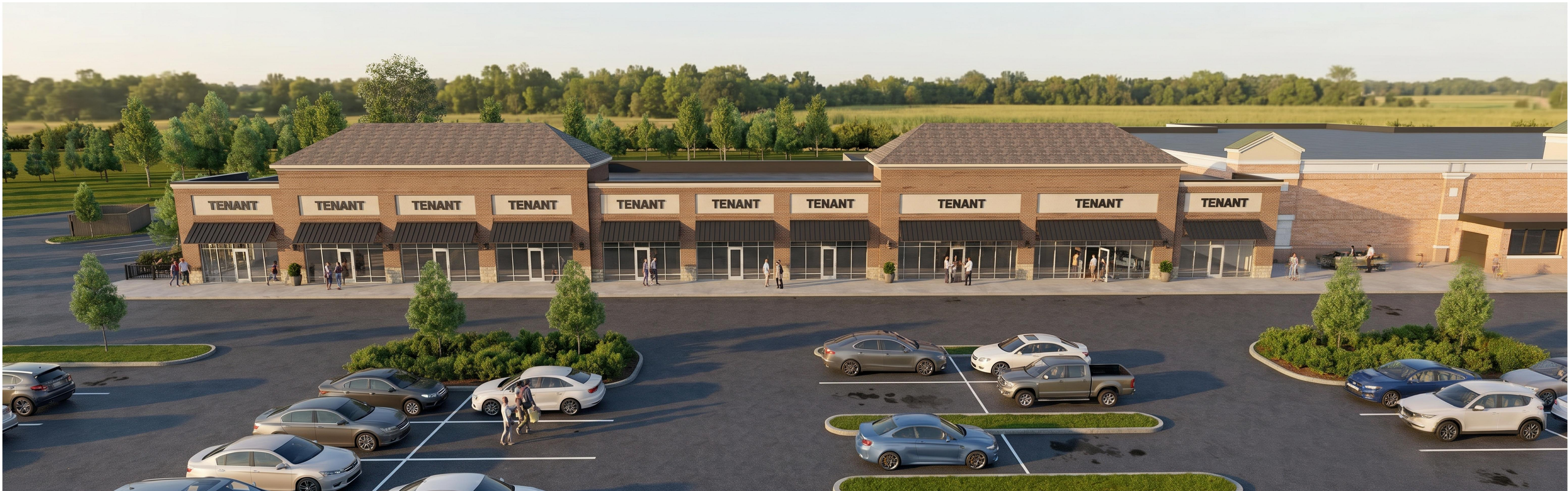
AERIAL VIEW LOOKING WEST
