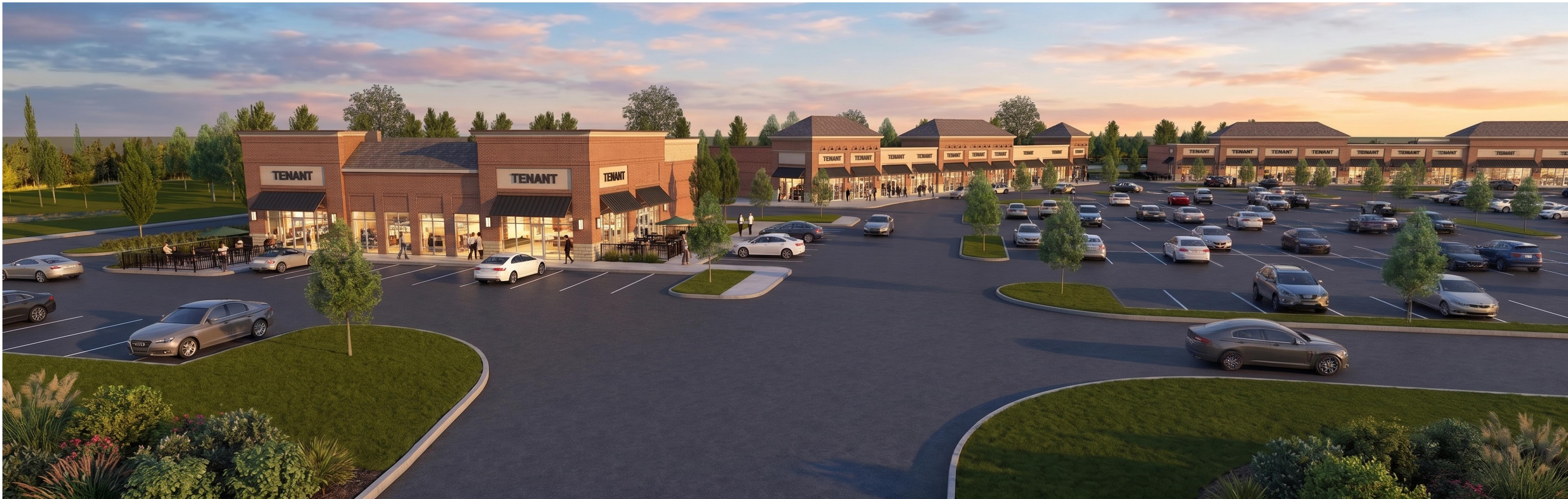
VIEW LOOKING SOUTHWEST
