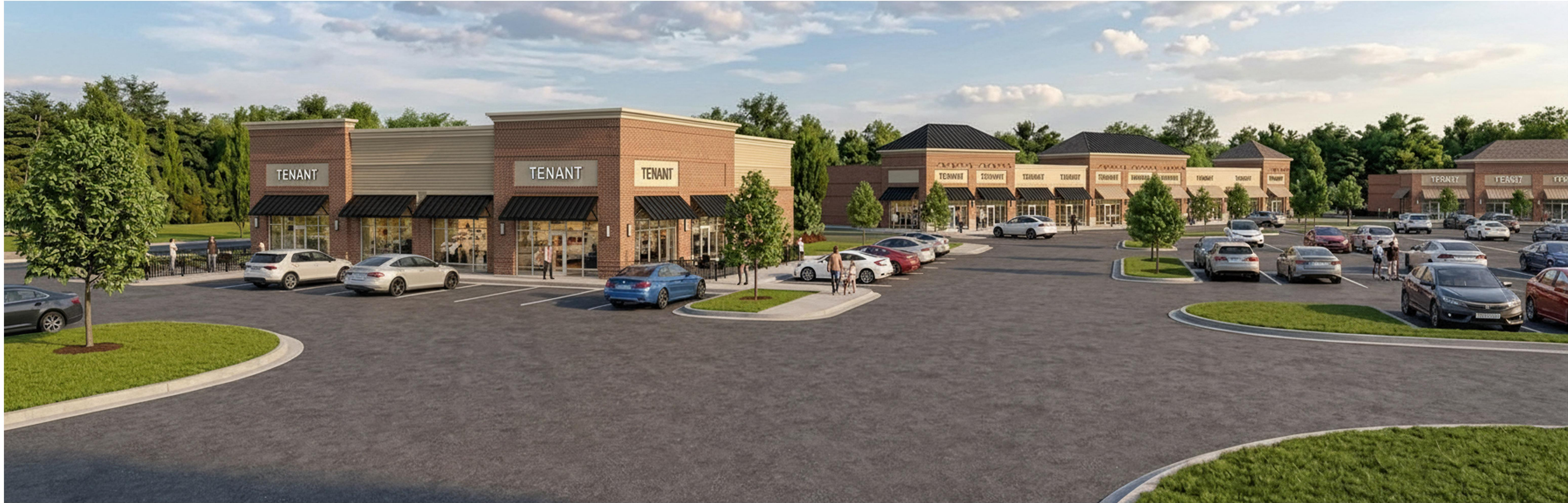
VIEW LOOKING NORTH
