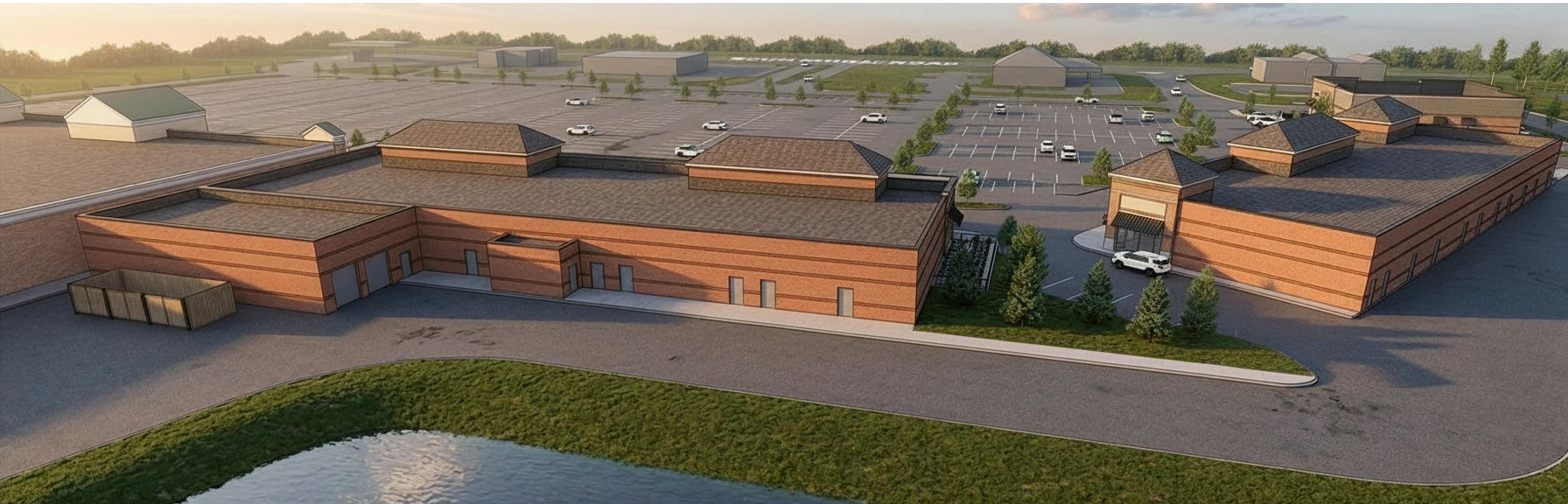
AERIAL VIEW LOOKING SOUTHEAST - JUNIOR ANCHOR REAR EXPANSION
