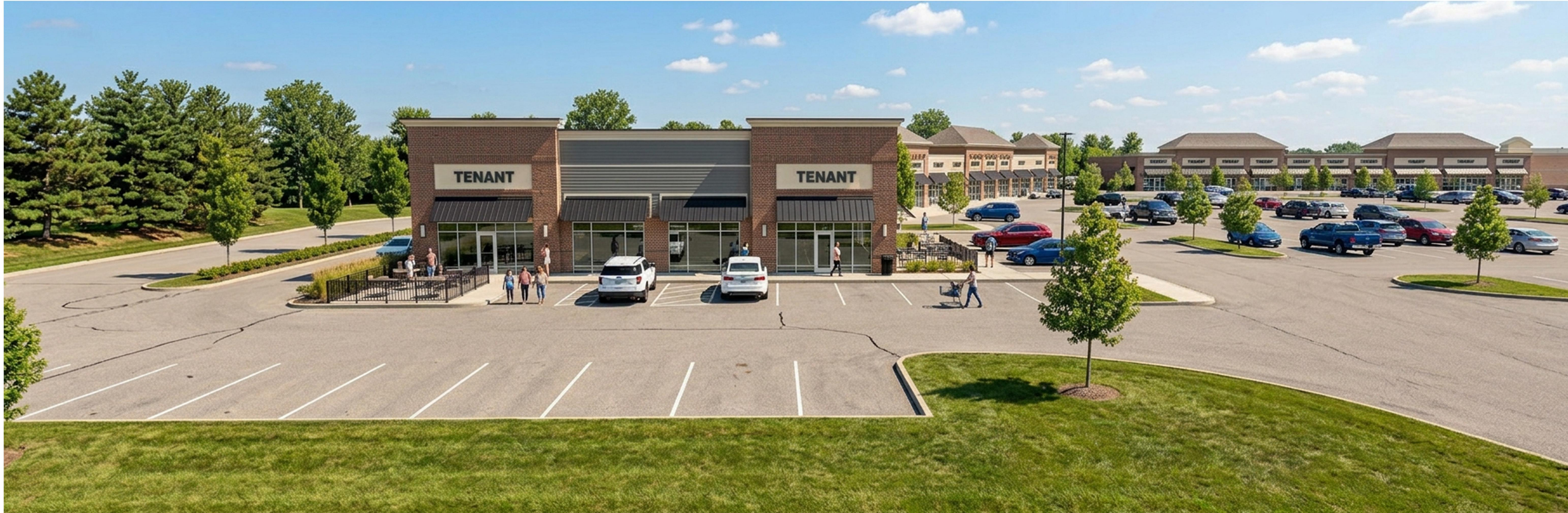
VIEW LOOKING NORTH
