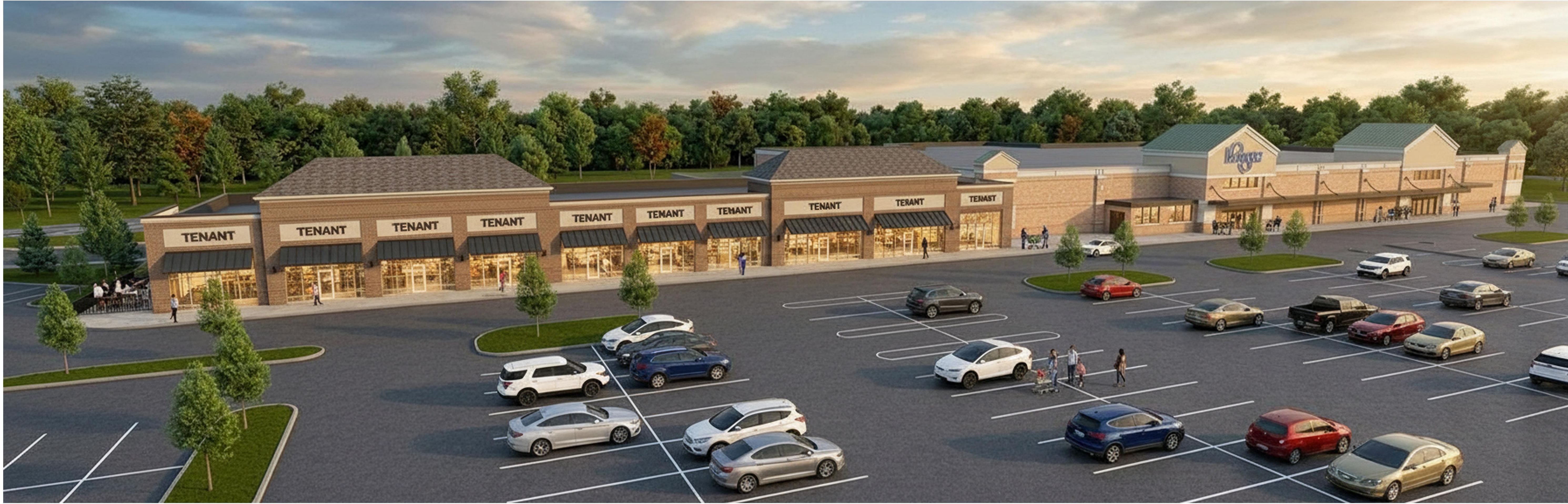
VIEW LOOKING NORTH
