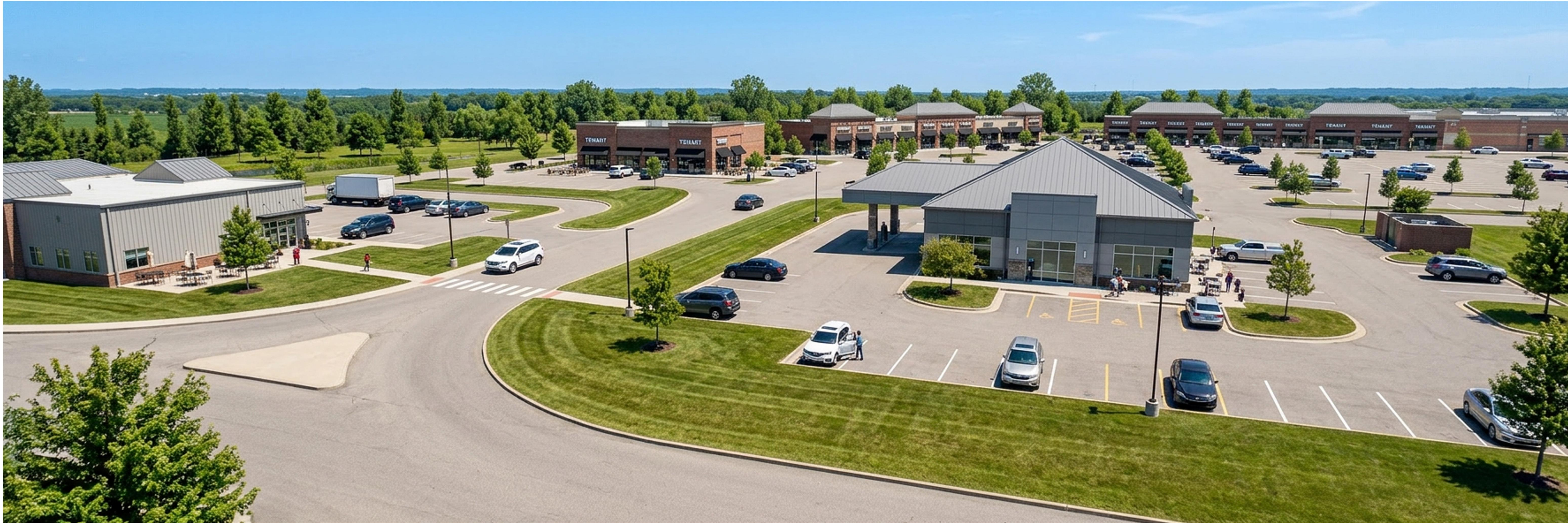
AERIAL VIEW LOOKING NORTHWEST
