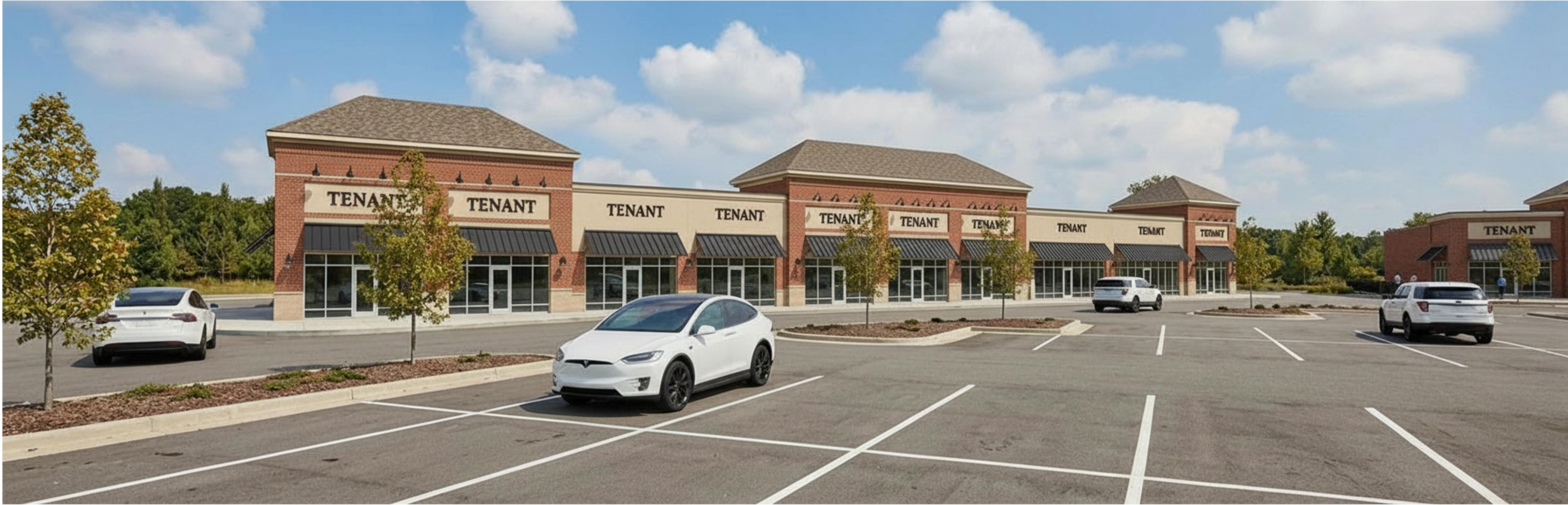
VIEW LOOKING NORTH
