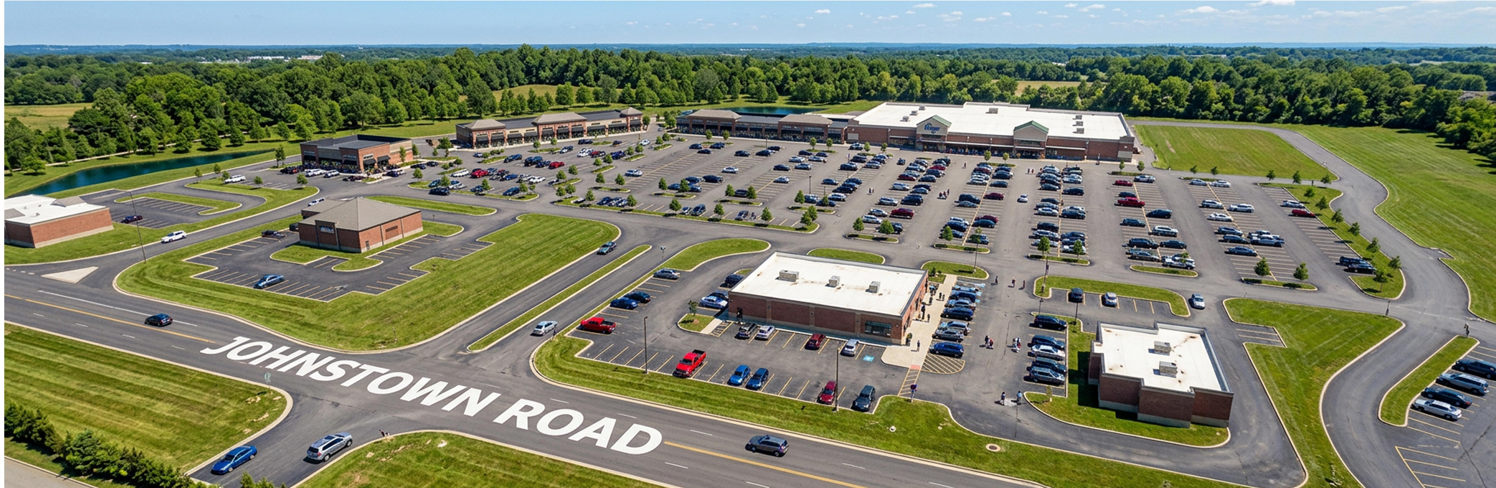
AERIAL VIEW LOOKING NORTHWEST
