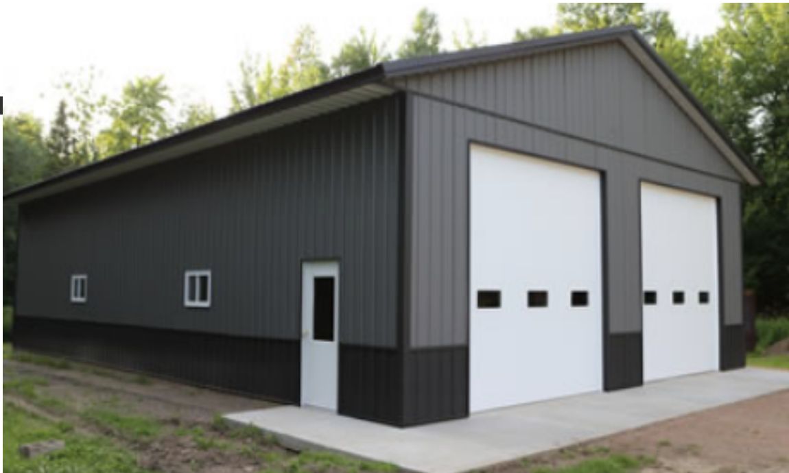
Example Image 3: Source - Steel Buildings Zone, www.steelbuildingszone.com
