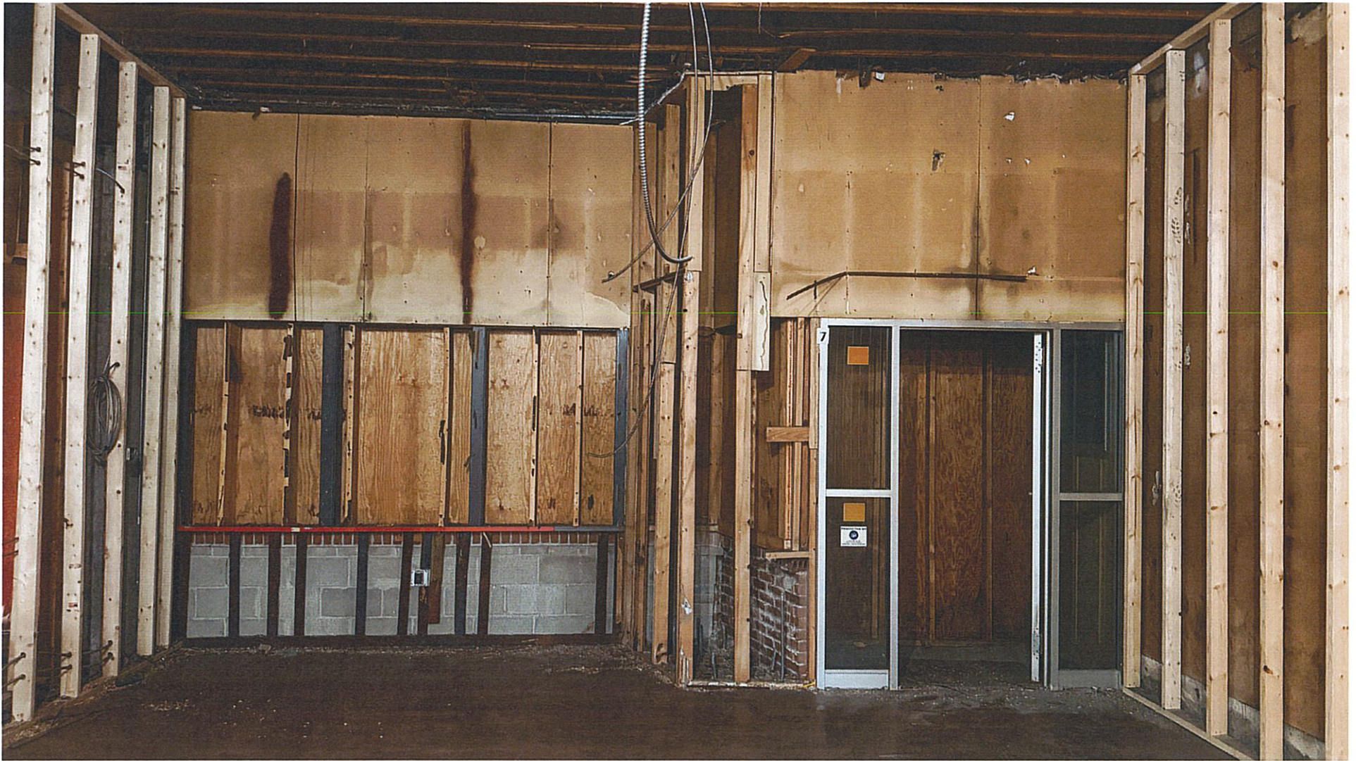
PHOTO OF EXISTING STOREFRONT FROM INSIDE OF WOOD PANELING
