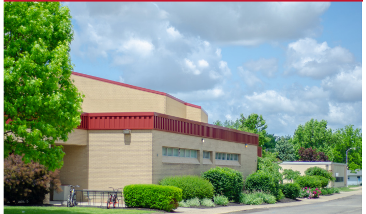
Figure 8.3: Johnstown Middle School
