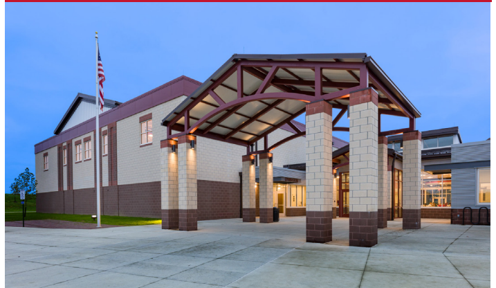
Figure 8.4: Johnstown High School
