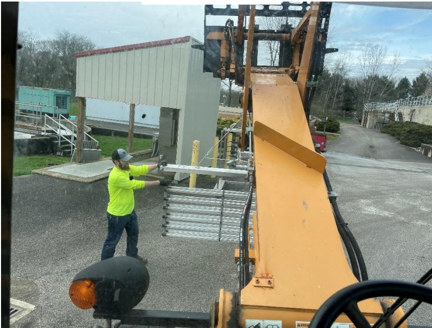
Installing UV Bulbs
