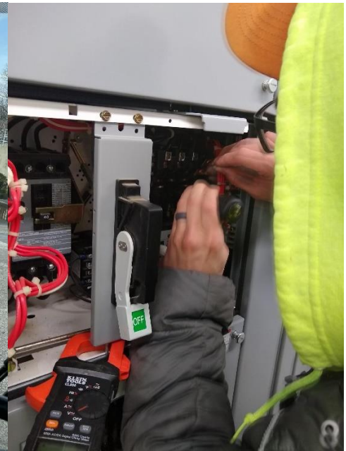
Contactor Diagnosis & Repair
