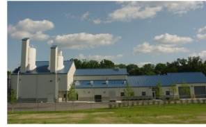
Versailles new 1.5 MGD lime-soda-ash softening WTP.
